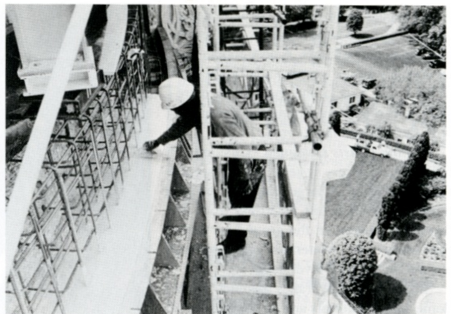
Technician finishes cast-in-place white quartz soffit and dentil section. A later placement of grey structural concrete will encase the epoxy coated reinforcing steel that ties the soffit and structural repair into the remaining original concrete.
