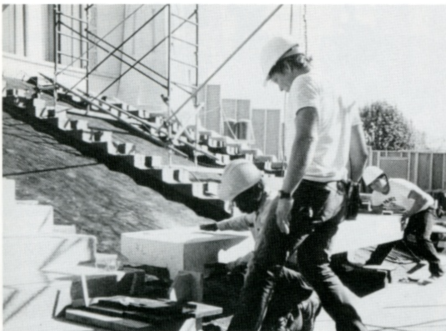
Workmen replace pre-cast stairs at entrance to the temple. A waterproofing membrane on the sloping concrete deck below the stairs protects occupied space inside the building.
