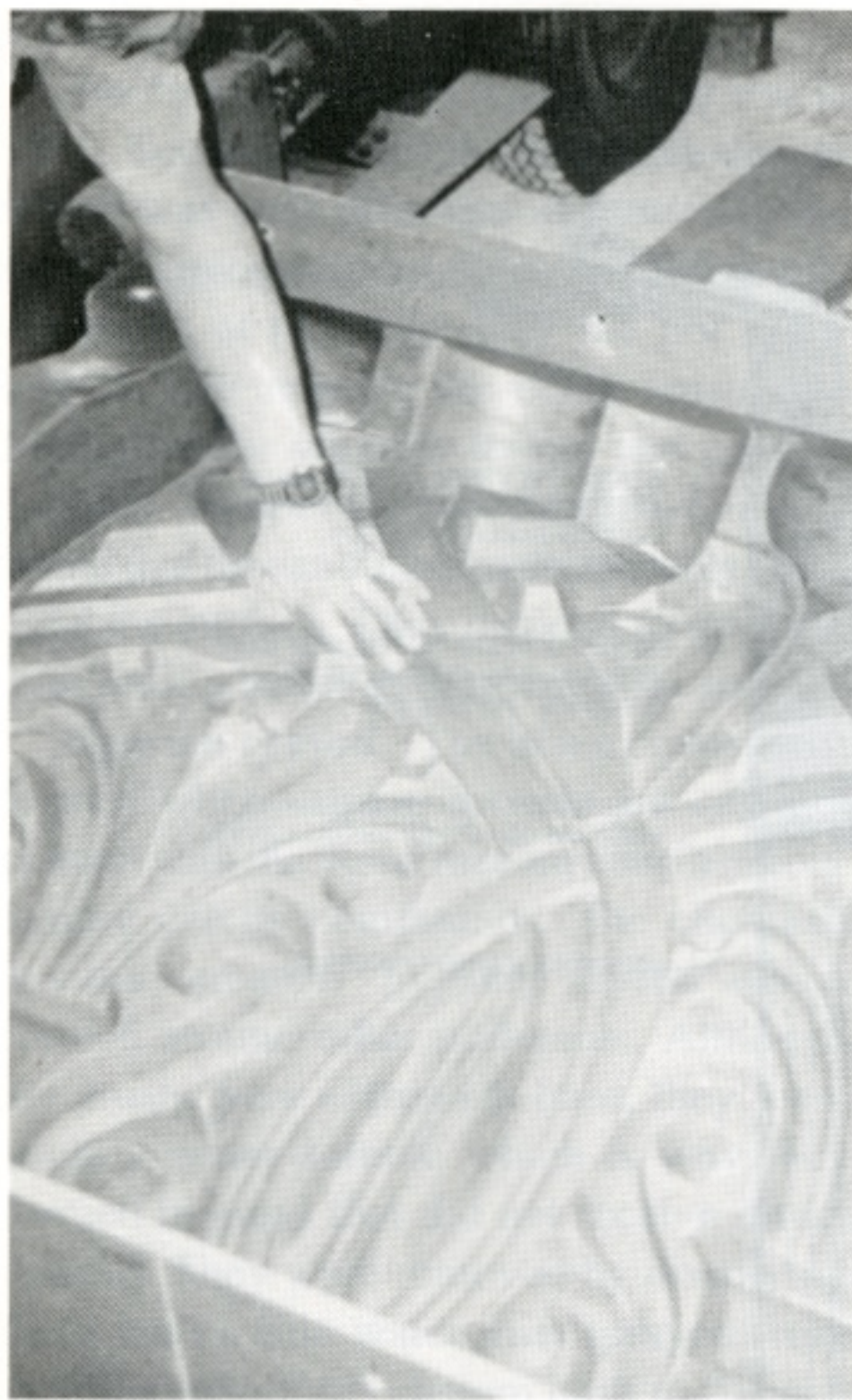
(Left) Intricate multi-piece fiberglass and rubber molds provided for accurate and efficient repair of the highly sculpted ornamental concrete components. (Right) Diagram by Wiss, Janney, Elstner Associates, Inc.
